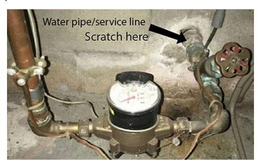
If the pipe is copper colored, and the magnet won't stick to the pipe, select "Copper" on the survey.
